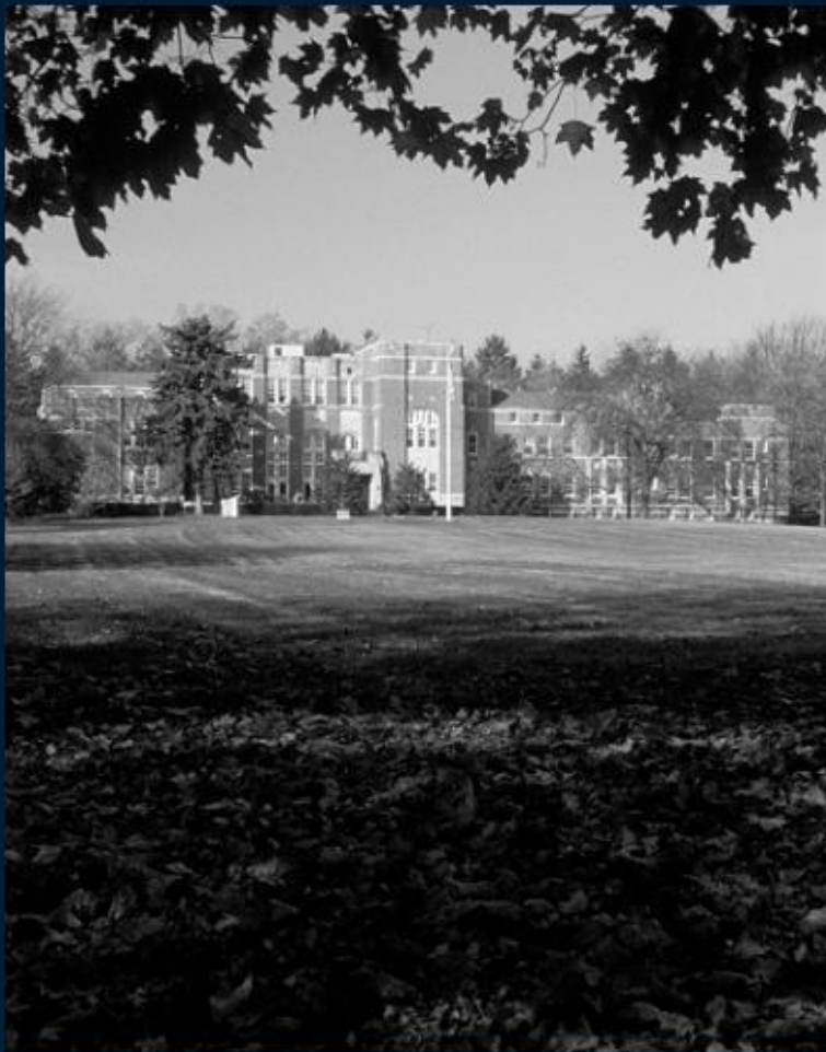
TS in America Headquarters - Rogers Building
